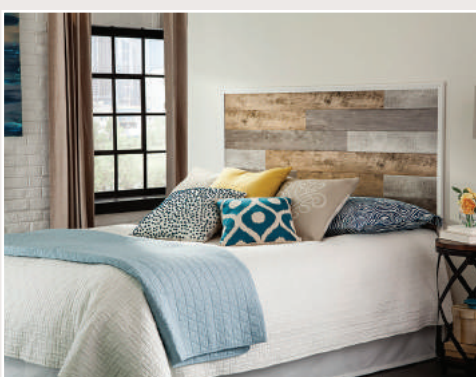
Headboard installed with construction adhesive.
